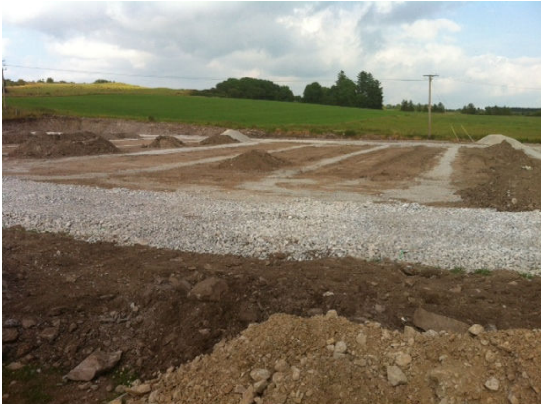
Stone base laid for track
