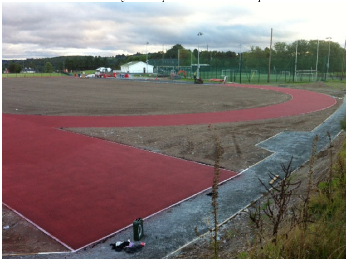
The walkway around the facility is also nearing completion
