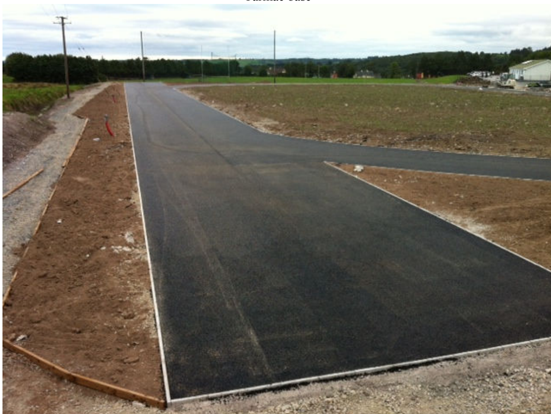
Track ready for next layer of rubber
