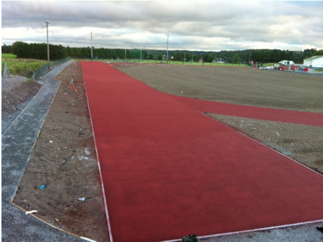
Track starting to take shape and infield is also landscaped
