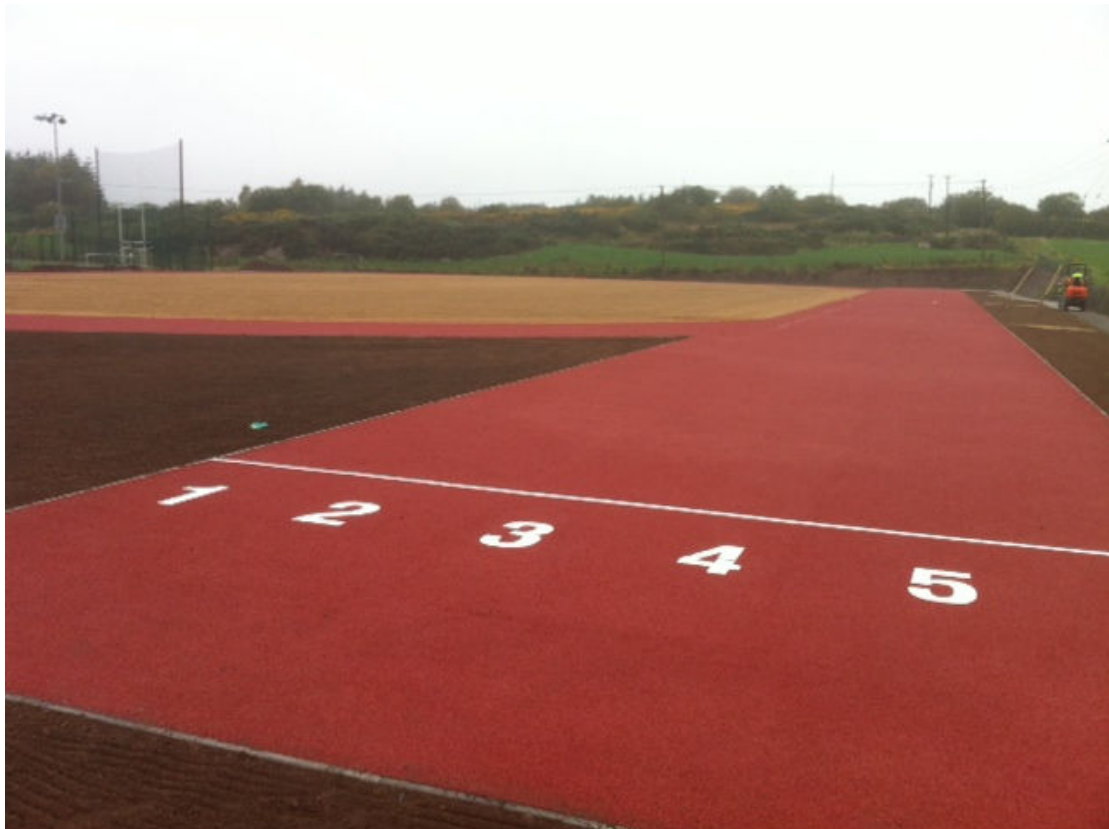
Lining of track begins
