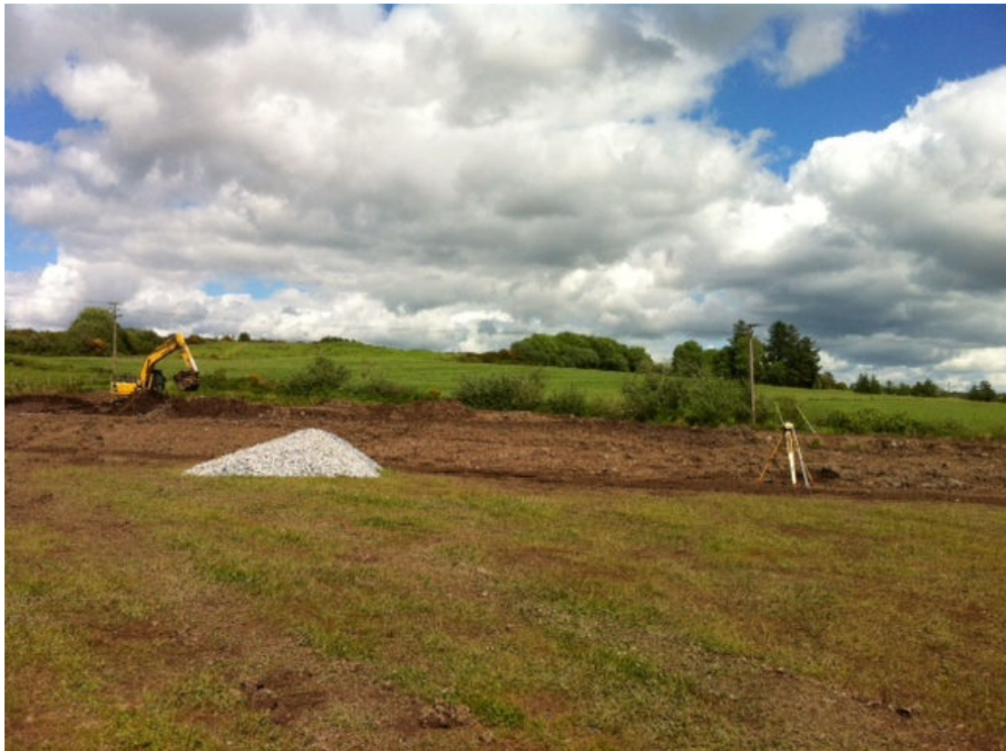
Ground work starts June 2013
